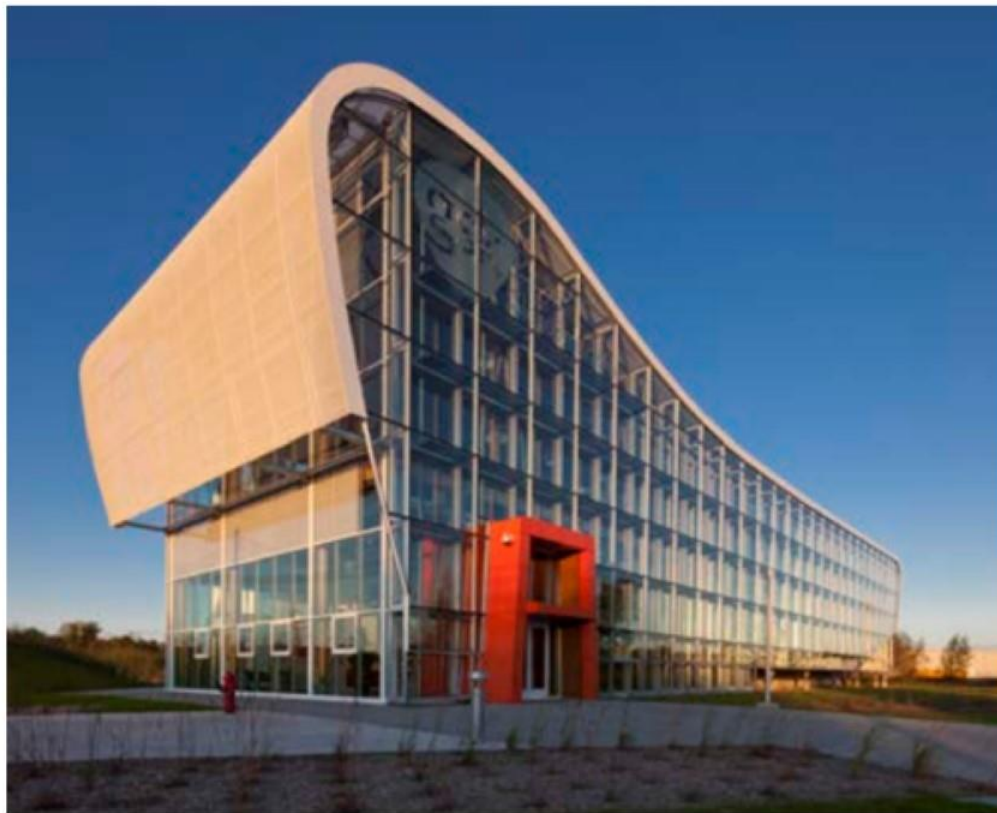
Nordic Structure's FSC-certified engineered timbers in new GlaxoSmithKline offices in Québec. Photo by Stephane Groleau.
